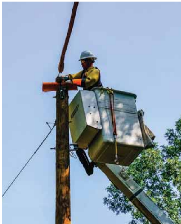
Journeyman Lineman Kaiden Davis working on a line in rural Pike County.
