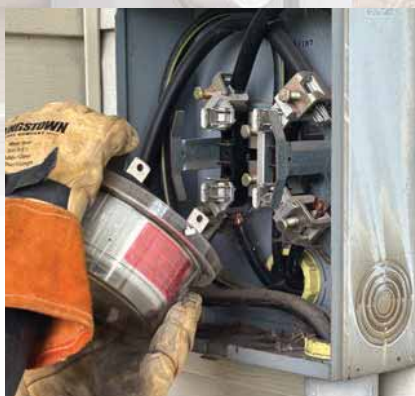
2-Remove Old Meter
