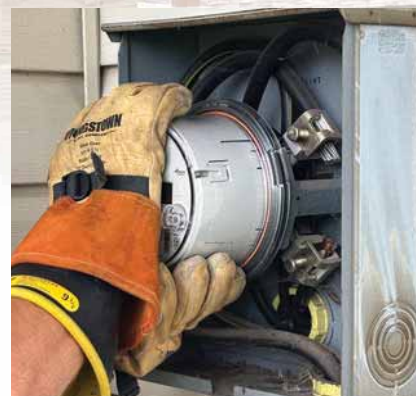
3-Install New Meter
