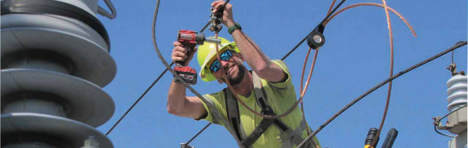
Harvel Substation: Line Foreman Shane Norris relocates a line to facilitate Ameren's metering upgrade
