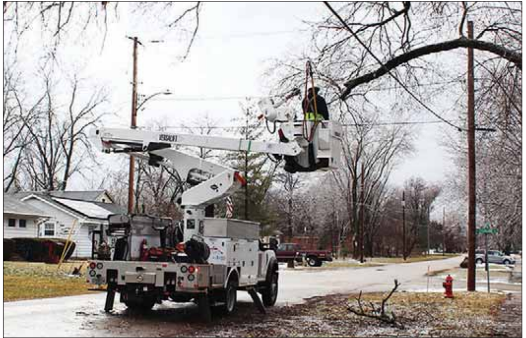
A Rock Energy crew work on getting branches off of power lines. The branches were coated with ice from a storm in February 2023.
