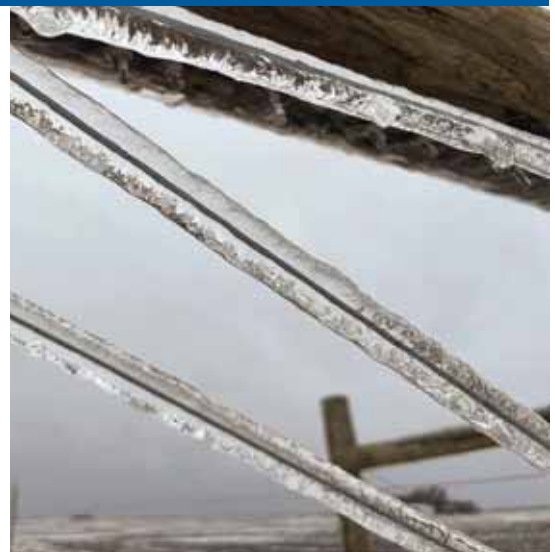
The Jan 22 storm complicated travel but didn't produce enough ice to affect operations. Utility poles and power lines are incredibly strong but unable to withstand two or three inches of ice when accompanied by strong winds.
