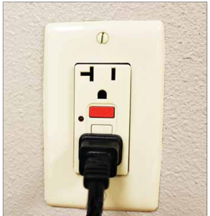
Using surge protector strips (above) can help keep your electronics from being damaged in the event of a power surge. Below is a ground fault circuit interrupter (GFCI), which helps to prevent electric shock and fire near sources of water.
