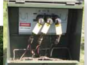
A field technician opens a green box as part of the underground residential distribution inventory. Warning signs are required on the outside, and danger signs are located inside.
