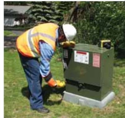
A field technician opens a green box as part of the underground residential distribution inventory. Warning signs are required on the outside, and danger signs are located inside.
