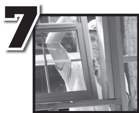
7 New replacement windows
