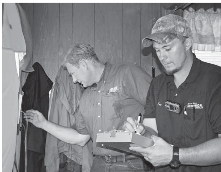
Spoon River Electric Cooperative Manager of Line Clearance Josh DeWees, also a BPI-certified energy auditor, provides Spoon River Mechanical Services Building Performance Analyst Joe Hedges blower door readings for calculations about the air loss in a customer's home.
