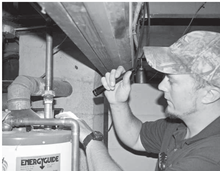
Spoon River Mechanical Services Building Performance Analyst Joe Hedges begins a safety check of a water heater before beginning an energy audit at a customer's home.
