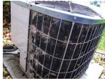
Cleaning off your air conditioner will not only make it run more energy efficient, it could also save money on your energy bill.
