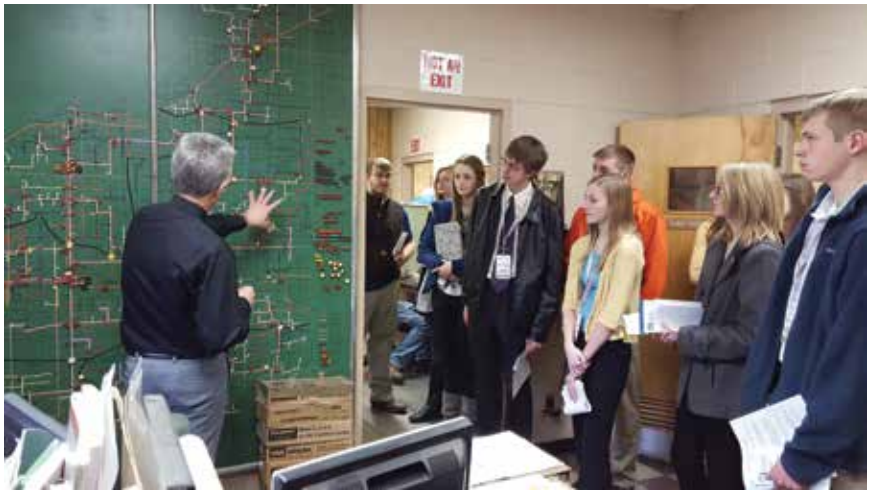
Tommie showed the students an overall view of our system, showing line breakers, capacitors, regulators and associated equipment. Even though this green board has been around since the 1950's, it provides a useful overview of our system.
