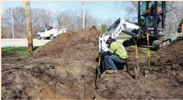
Rock Energy Cooperative natural gas crews—Gas Technician James Gander in the excavator and Apprentice Gas Technician Dan Alseth on the ground—are working in Rockton to replace old gas mains. The project will continue throughout the summer.
