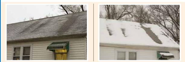
Are your shingles shimmering with frost? Great! Frost (or the lack thereof) can be an indicator of how attic insulation is performing. Bare spots may mean insulation has fallen or holes/gaps exist. Even small gaps in the insulation can create space for heat to escape out your roof. Check your roof the next time there is adequate frost or light snow on it.
