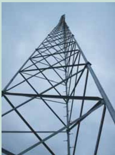
Towers, like this 180-foot tower near Stewardson and Strasburg, are popping up around Shelby Electric's service territory as PWR-net wireless broadband expansion continues.
