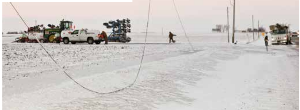
A Shelby Electric Cooperative crew, with assistance from a Jackson Purchase Energy Corp. crew from Paducah, Kentucky, repairs a line brought down by ice and wind near the Findlay-Assumption blackout. ▶
