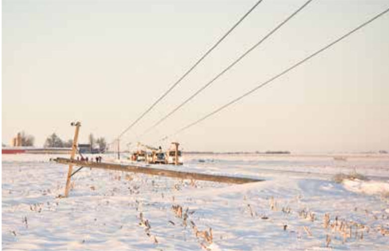
A Shelby Electric Cooperative crew, with assistance from a Jackson Purchase Energy Corp. crew from Paducah, Kentucky, repairs a line brought down by ice and wind near the Findlay-Assumption blackout. ▶
