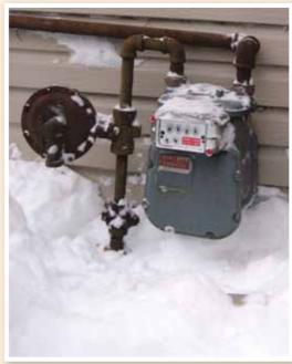
As you're shoveling sidewalks and driveways this winter, remember to check your natural gas meter and pipes for drifted snow, top, which can cause problems. When exposing the meter and pipes, avoid using a snow blower. Instead, gently remove snow and ice from the area.
