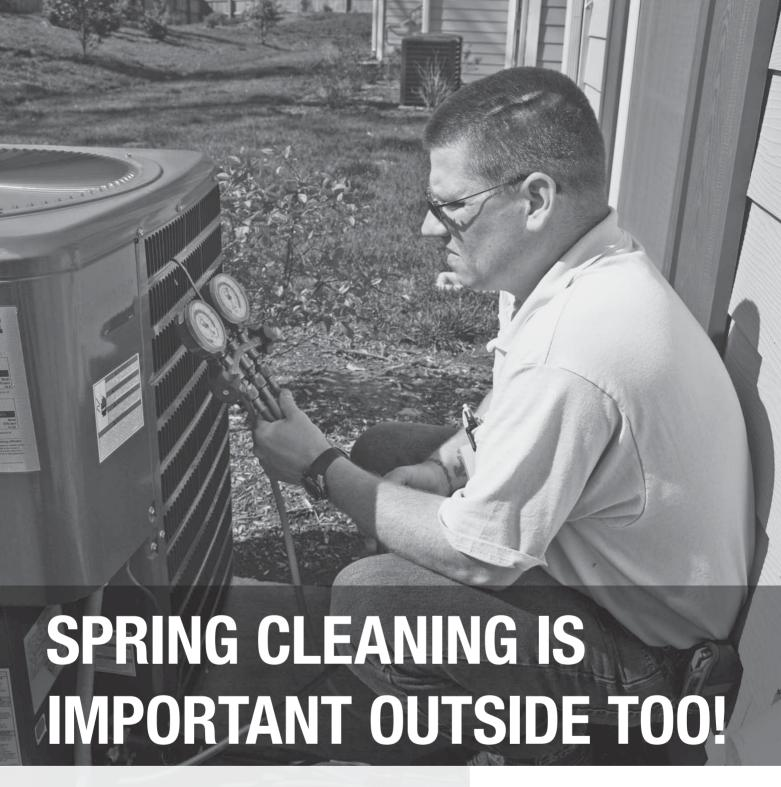
Making sure the coils on your air-conditioner or heat pump are clean helps reduce energy consumption and reduces equipment failure. Having a professional technician perform a regular 'check and clean' can ensure your cooling system works at peak efficiency. Make sure the electricity to the unit is turned off before performing any maintenance tasks.
