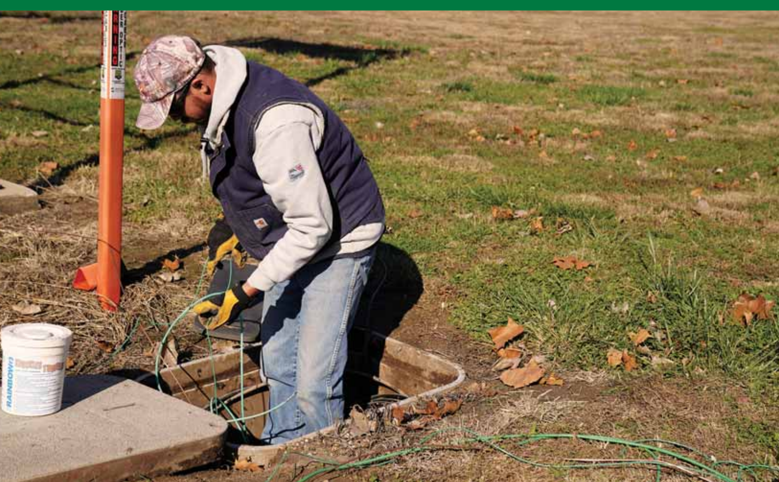
Internet Technician Drew Klingele working on a fiber drop in Hardin.
