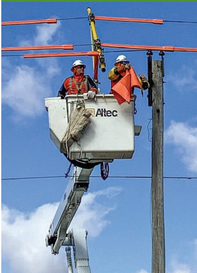
Linemen Mitch Stanciu (left) and Brock Cook
