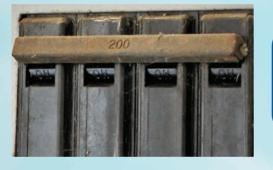
If that does not work, check the breaker located under your electric meter. Do not touch the meter or use any tools; the breaker should be easily accessible by hand. Never go near a downed power line and don't stand in water while touching electrical equipment!
