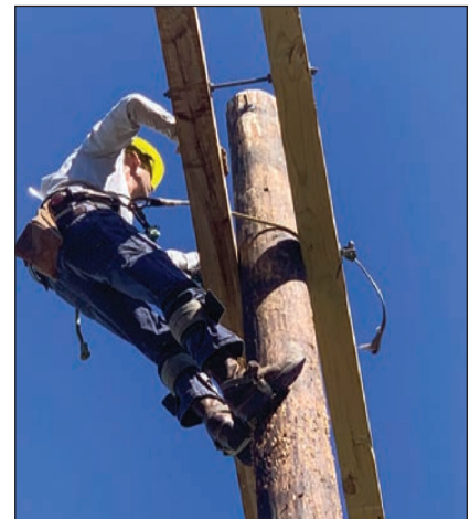
Construction Superintendent Brian Chevalier finished third overall in individual event scoring.
