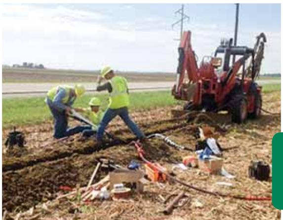
*RECC linemen splice connections between two reels of underground wire, which each hold 2,500 feet of cable. Grounding grids are also connected every 1,200 feet along the cable installation.*
