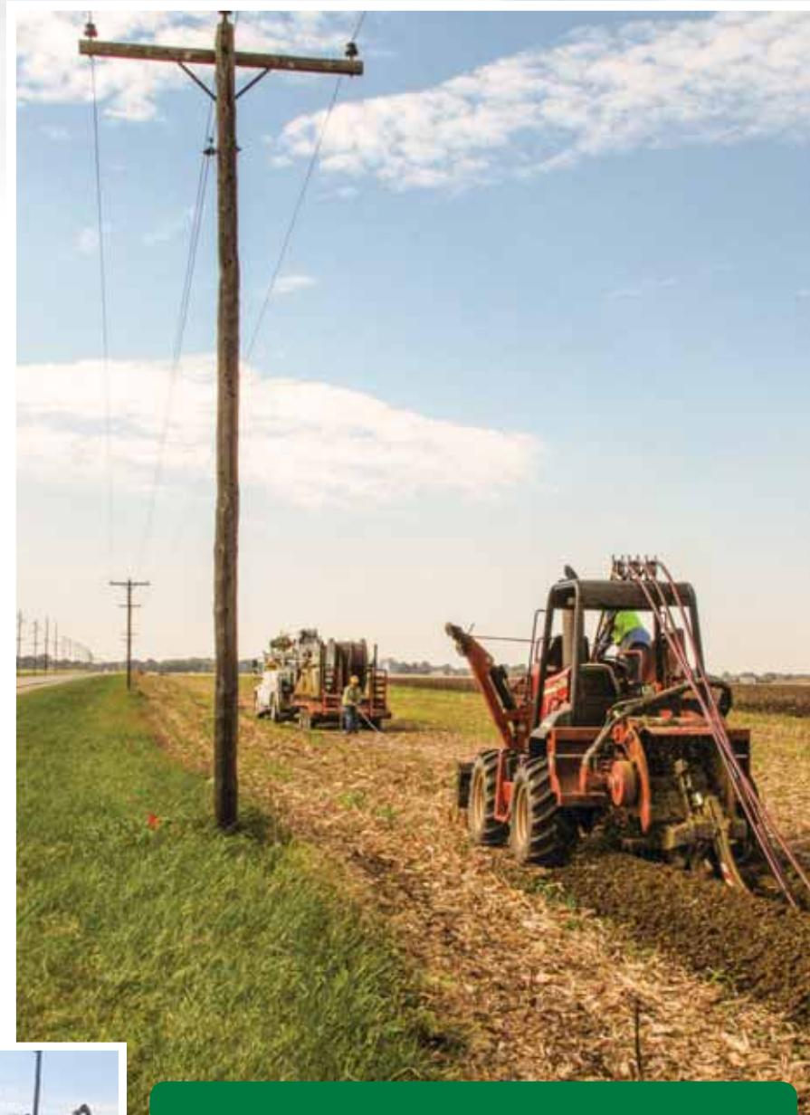
*New three-phase cables are trenched along State Route 104 east of Auburn, to replace 2.3 miles of deteriorated overhead lines.*
