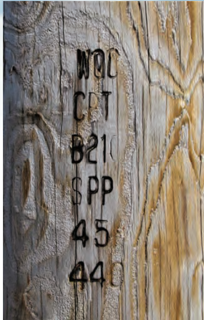
Birthmarks can be easily seen on new poles but become less visible over time, which is illustrated above.
