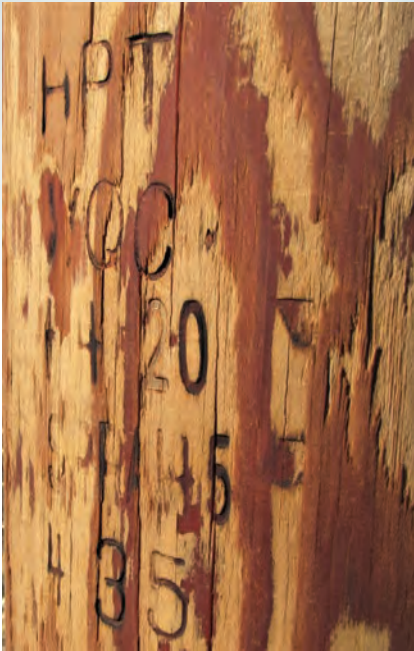
Birthmarks can be easily seen on new poles but become less visible over time, which is illustrated above.
