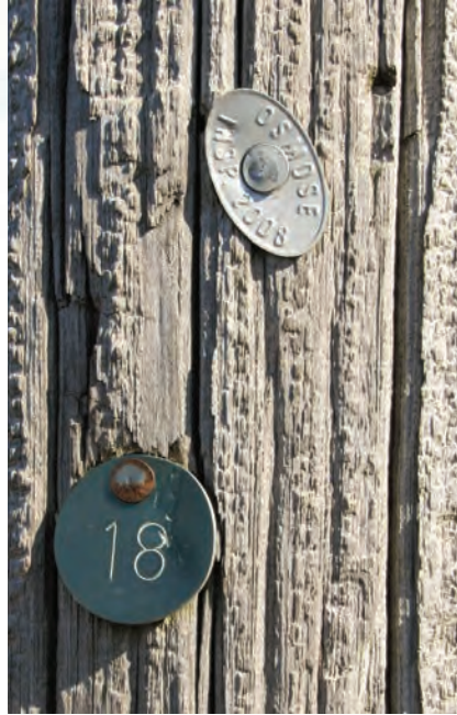
Inspection tags from 2008 and 2018
