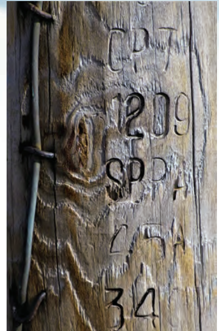
Birthmarks can be easily seen on new poles but become less visible over time, which is illustrated above.
