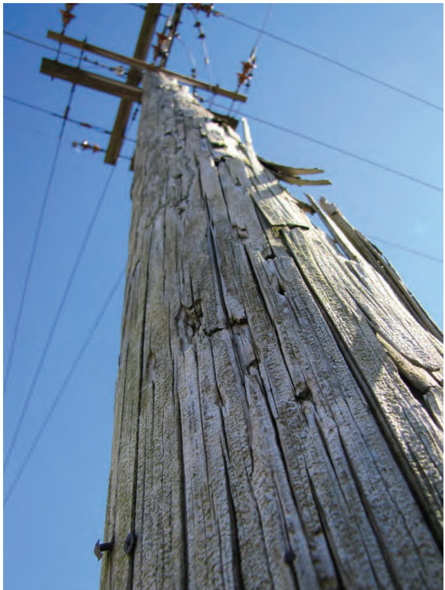
This three-phase pole has weathered many storms. Notice the lineman's hook marks.
