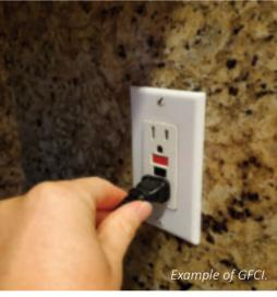
GFCIs constantly monitor current flowing through a circuit. If the current flowing into the circuit differs by a small amount (even as small as 4 or 5 milliamps) from the returning current, the GFCI interrupts power to prevent shock or injury. However, GFCIs only do their job when they are in good working order: test them each month to be sure.
