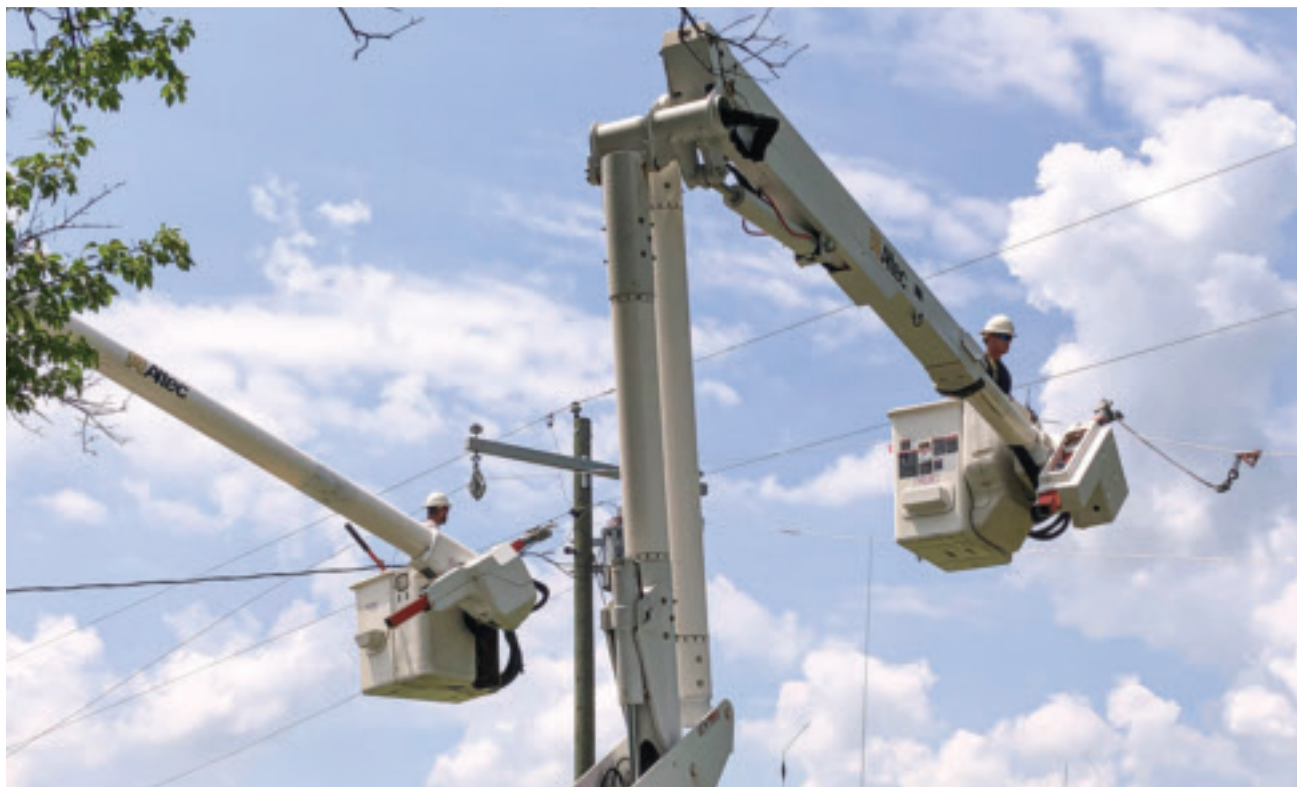
The heat of summer hasn't slowed down the EnerStar crews. The co-op is busy rebuilding about 7.5 miles of 3-phase line just east of Kansas, IL.
