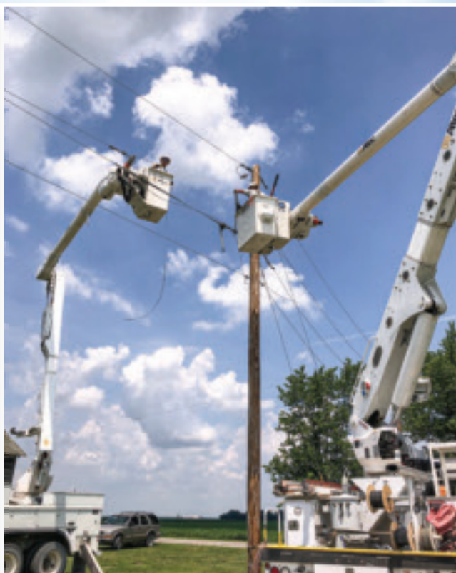
The heat of summer hasn't slowed down the EnerStar crews. The co-op is busy rebuilding about 7.5 miles of 3-phase line just east of Kansas, IL.
