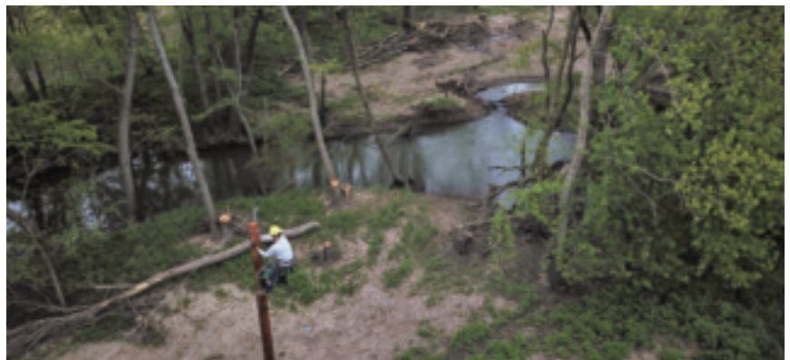
▲ Drayton Davis, Apprentice Lineman
