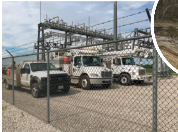
Since March, the underground crew has been starting and ending their days at the Old State substation to do their part in preventing the spread of the COVID-19 virus.
