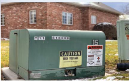
work during an outage and create a serious safety hazard. We need a minimum of 10 feet of clearance in front of the transformer (the side that is padlocked), as well as ample clearance on the other three sides.
