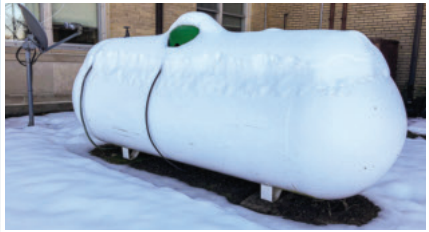
Keeping your propane tank free from snow and ice will allow your propane provider safe and easy access to service your tank.
