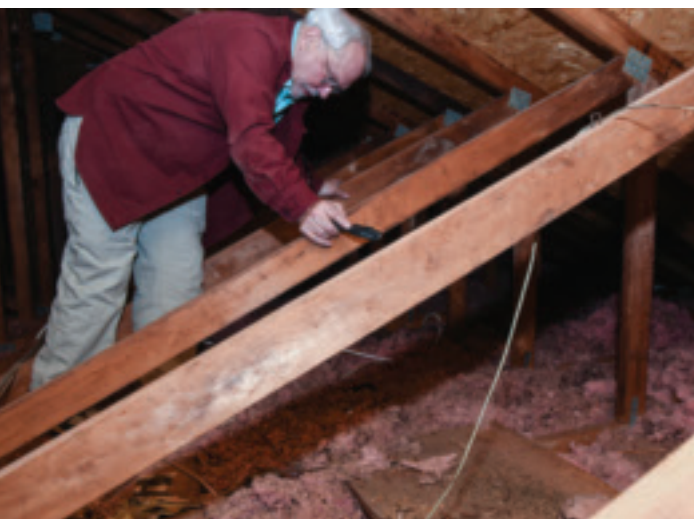
Your attic can be one of the greatest sources of heat loss in your home. An energy auditor can look for issues and recommend steps to correct them. Photo credit: "Auditor inspects the attic" by Andy Harper (CC BY-NC 2.0)
