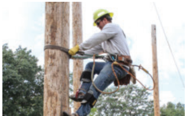
Apprentice Dalton Brown placed third in the individual apprentice H-structure event.
