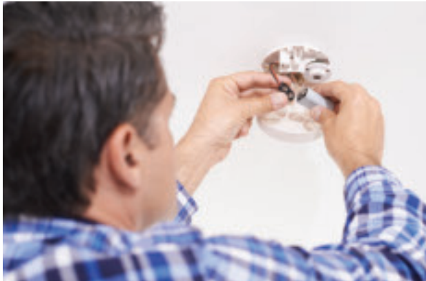
On November 3, daylight saving time ends. While you are changing your clocks, do not forget to change the batteries in your smoke and carbon monoxide alarms.
