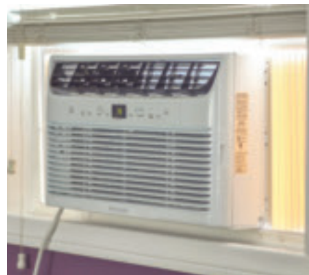
Make sure your window A/C unit is installed flat or according to manufacturer's directions, so that it drains properly. Photo credit: Your Best Digs
