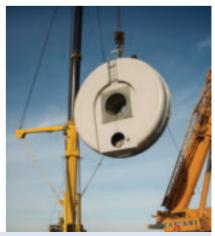
Nacelle being placed on the 230-foot tower, followed by the 62,000-pound generator; 85-foot blades complete the installation
