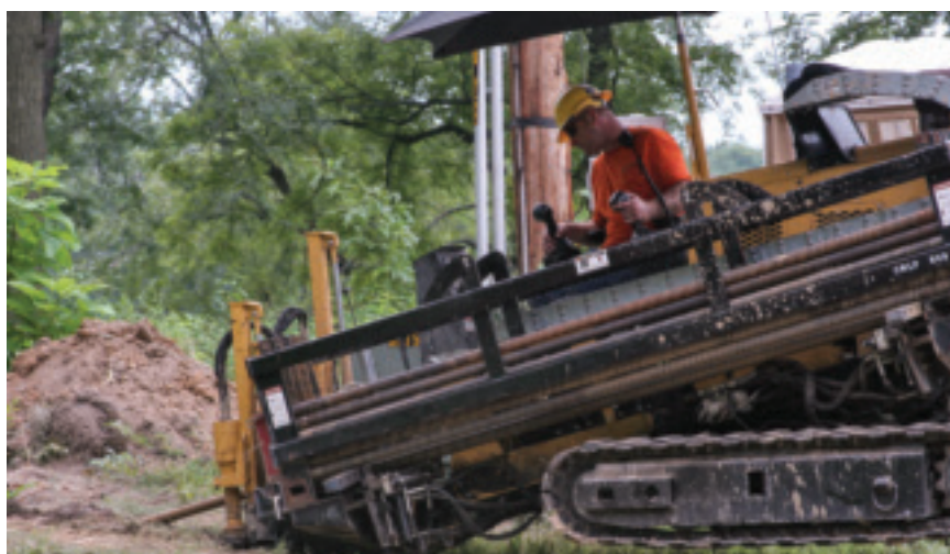
Installation of a closed-loop geothermal system.
