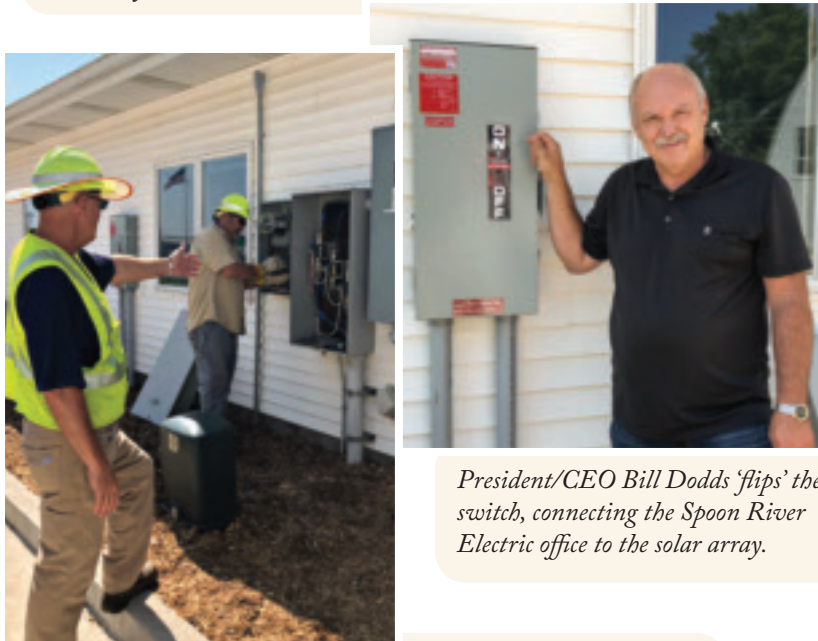
Ameren linemen switching out our old meter to the new net meter, which reads what the solar array produces and what the office electric usage is all at the same time.
