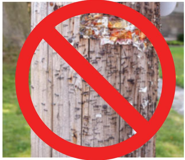
Utility workers are sometimes tasked with climbing those same utility poles to work around power lines that carry 7,200 or more volts of electricity. Foreign objects such as staples or nails embedded in the pole can damage a utility workers gloves. Those gloves are meant to insulate workers from high voltage and protect them from being electrocuted.
