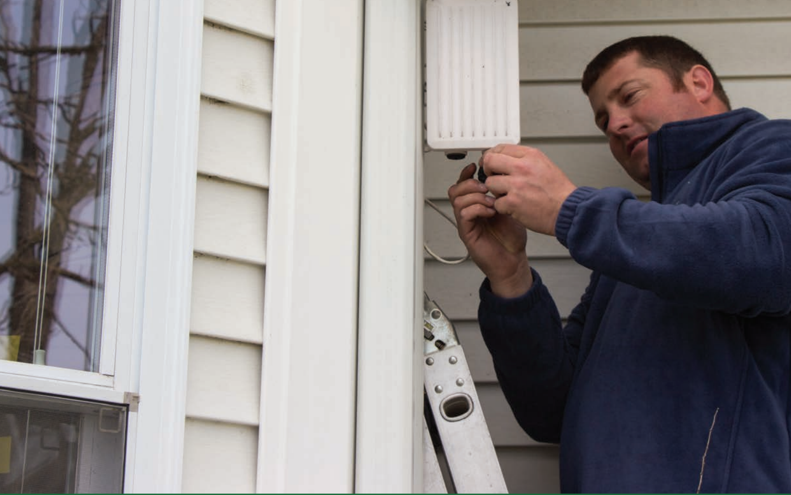
Lance Ridenour working on a wireless internet installation.
