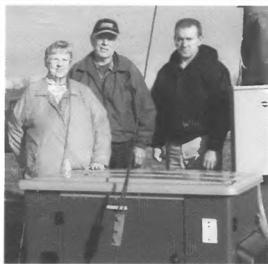
Helen and Bob Meers worked with Member Services Coordinator Tim Bohnhoff to purchase and install their new home generator system.
