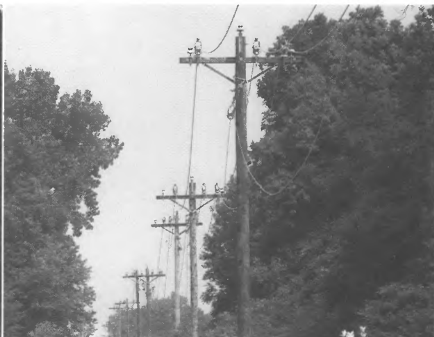
▼ New three-phase line pulled in on rollers
