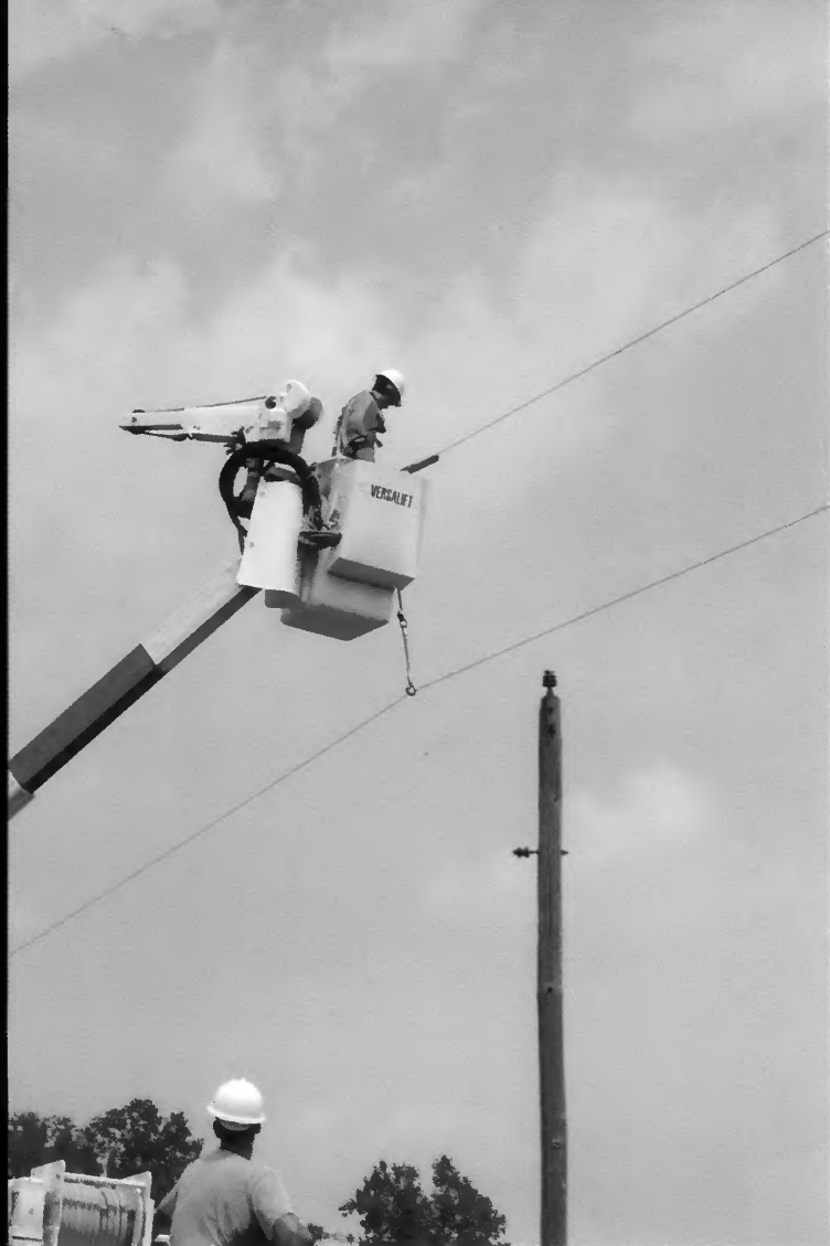
Zachary Vedder, Apprentice (above in the bucket truck and picture below), takes the single phase line off the pole so the pole can be replaced and the customer does not lose electrical service during the process.
