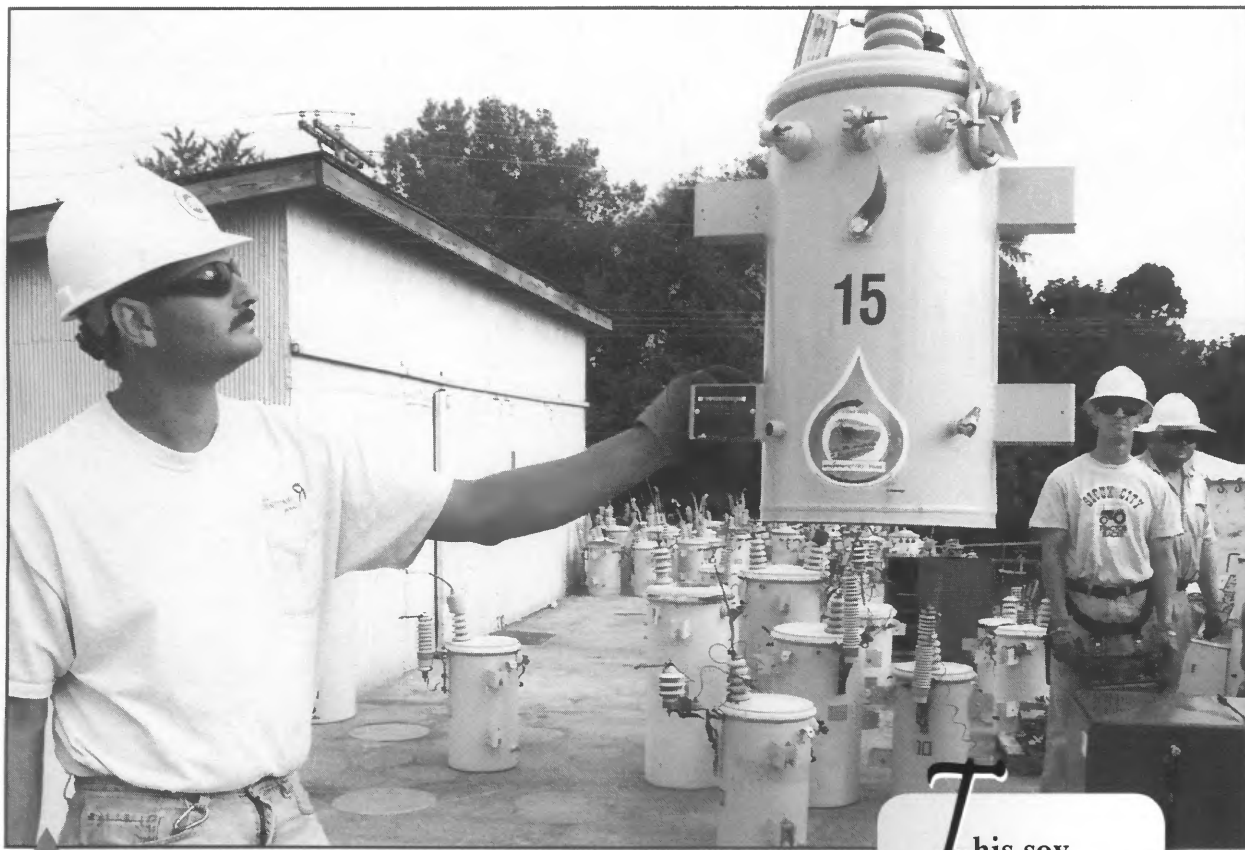
Journeyman Lineman Jeff Palmer (left) inspects one of the co-op's new soybean oil based transformers as Apprentice Lineman Allen Plott operates the lift and Journeyman Lineman Jeff Cates assists.
