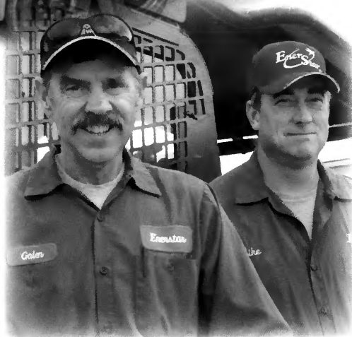
During November and December, EnerStar's Galen Satterfield (left) and Mike Huddleston have been clearing rights of way to improve system reliability.
