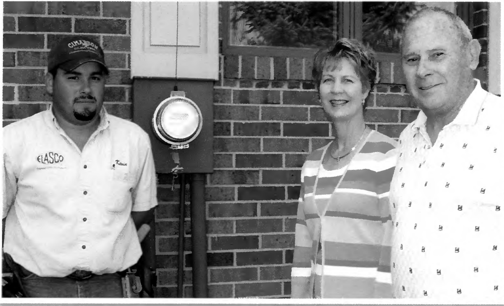
Kevin Tarr, AMR meter installer from Hughes Supply Company, and Jill and George Scott, recipients of the first AMR meter.
