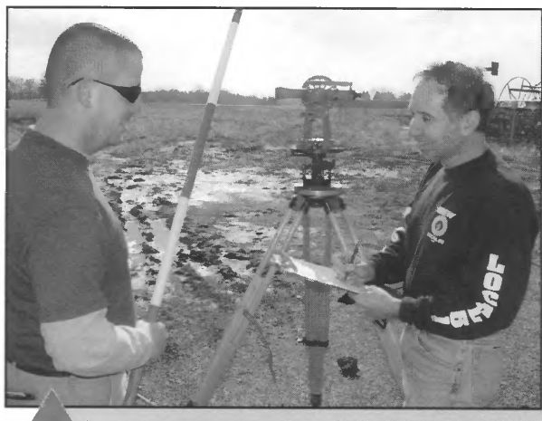
Jason Cotner, Assistant Field Engineer, (left) and Steve Wheeler, Field Engineer, survey a member's building site.
