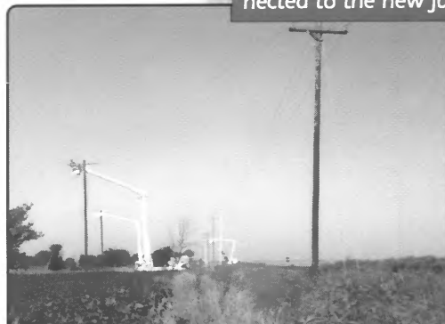
The new poles (left) being moved at the Meadow Slough Bottom.
