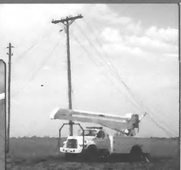
Wires waiting to be tightened or "sagged" (line crew term).
