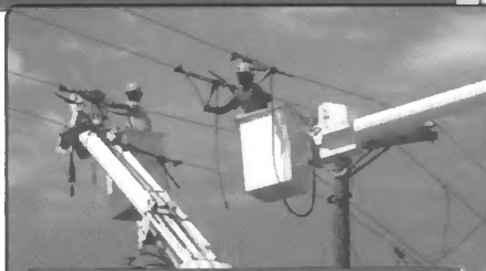
Making final adjustments to the new three-phase junction pole.
