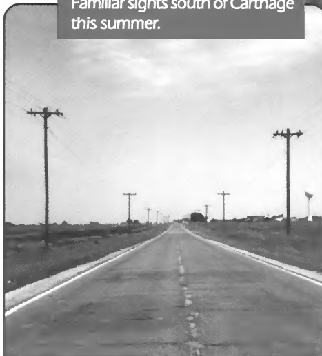
The lines on the left will be taken down to make room for the new road. The lines on the right are new.
