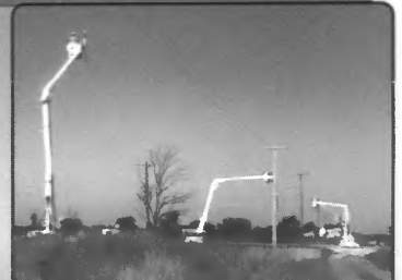
At this crossing, new wires were attached at the west end of the line with splices. Each phase, one at a time, was moved and placed on the new cross arms.
