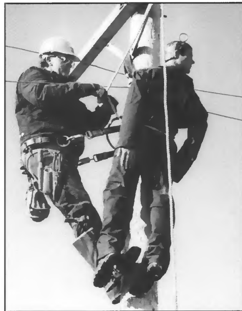
Foreman Bill Allen performs the annual pole-top rescue certification.
