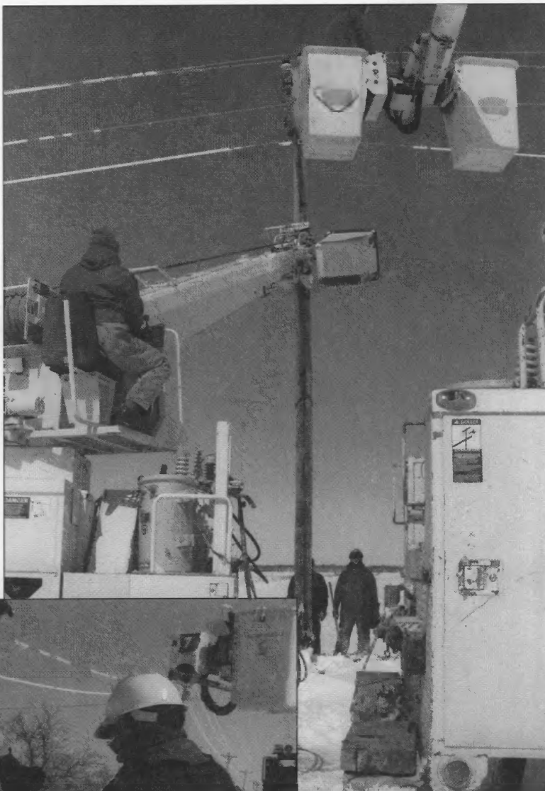
◀ A crew from Shelby Electric Cooperative, Shelbyville, changes out a broken pole.
