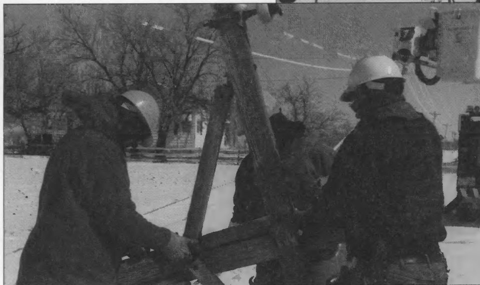
An EIEC employee ▶ puts hardware on a new pole.
