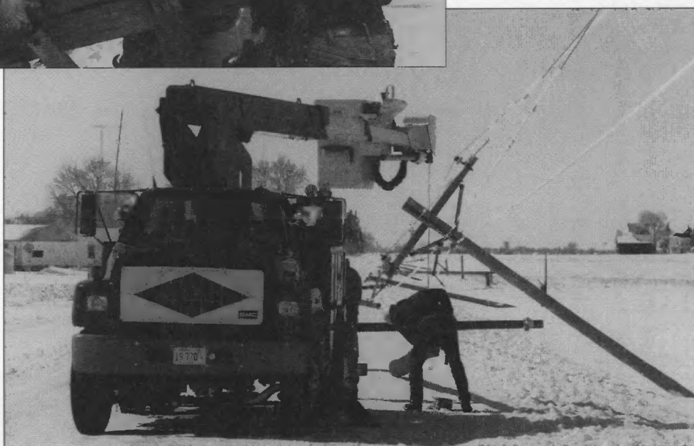
◀ A crew from Shelby Electric Cooperative, Shelbyville, changes out a broken pole.
