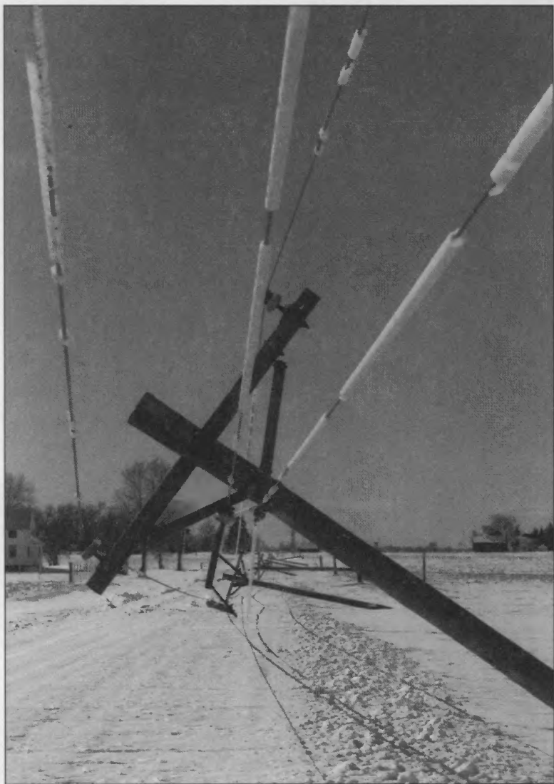
In a sight repeated all too often, a series of broken poles lies across a road. In all, some 120 poles were broken in the storm.
