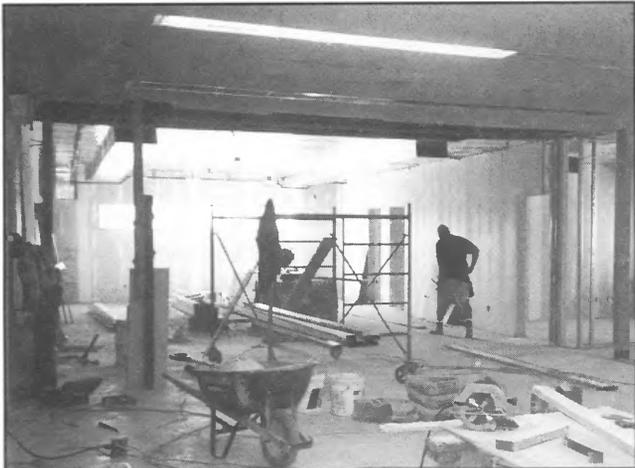
The original 1954 exterior block and brick wall totally removed in the new engineering spaces. Note the temporary braces holding up the juncture of the old and new roofs.
