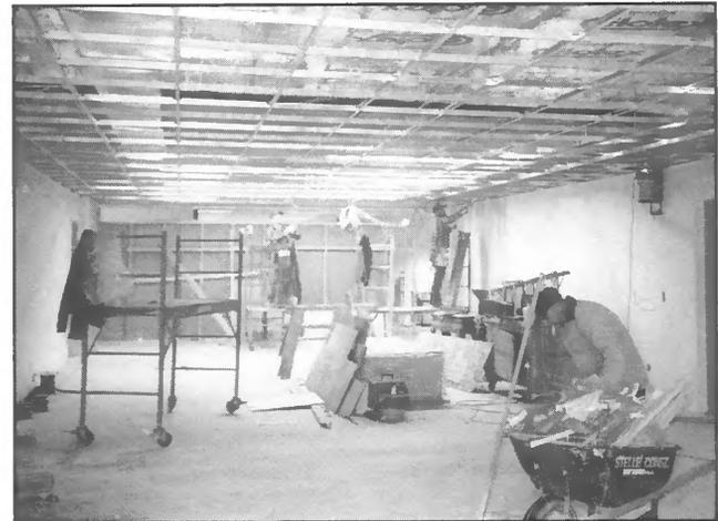
Closing in on the completion. Putting the dropped ceiling in the new engineering space.
