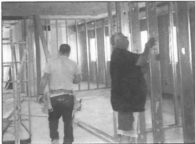
Installing the metal studs for the office walls in the new engineering department space.
