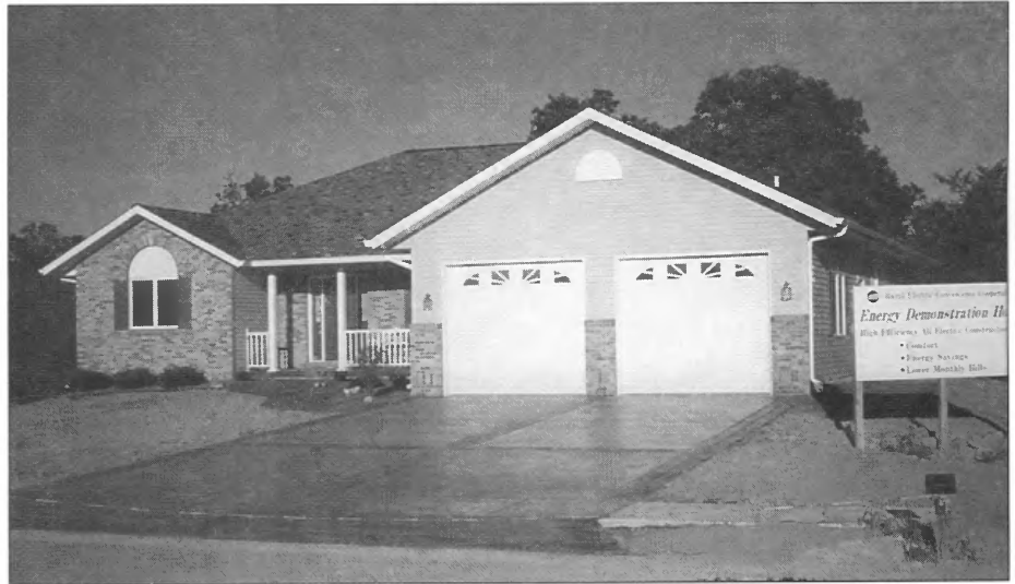
The Energy Demonstration Home looks like any other attractive new house, but energy costs may be as little as half of other "typical" homes.
