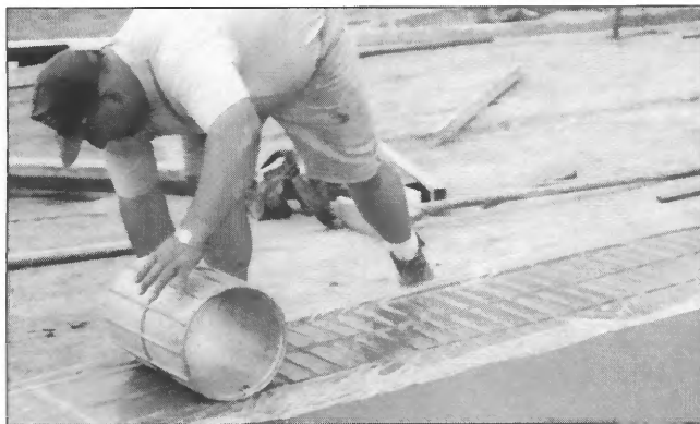
Steve Johnson rolls a brick pattern along the tinted driveway, one of the many extra touches built into the Energy Demonstration Home.
