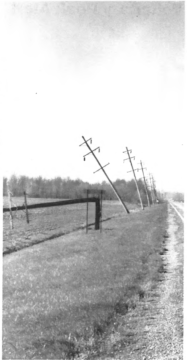
Clockwise from above: A pole leans across a road in front of a damaged farm: note the downed lines in the foreground. Another downed distribution line. A transmission pole with a distribution underbuild is broken off, while others lean.
