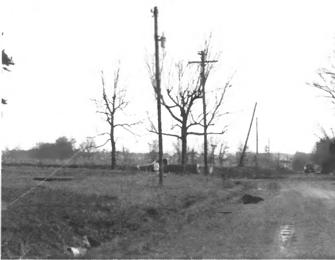
Clockwise from above: A pole leans across a road in front of a damaged farm: note the downed lines in the foreground. Another downed distribution line. A transmission pole with a distribution underbuild is broken off, while others lean.
